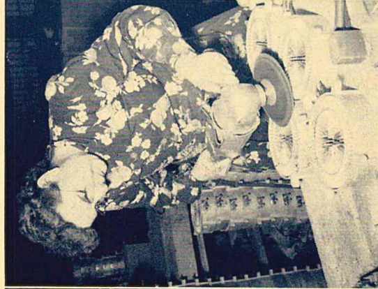
Mary Chamberlain finishing cast aluminum heating elements with a hand disc grinder.
